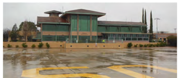
Terminal Viewed from Airside
