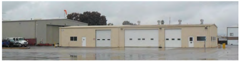
Unstaffed Fire Station
