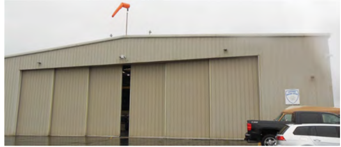
California Highway Patrol Hangar
