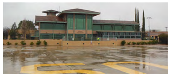
Terminal Viewed from Airside
