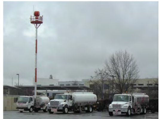
Airport Rotating Beacon and Mobile Refueling Trucks
