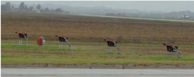
Precision Approach Path Indicator (PAPI-4)
