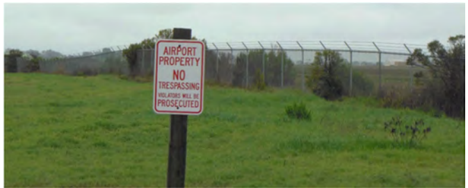
Security Signage and Perimeter Fencing
